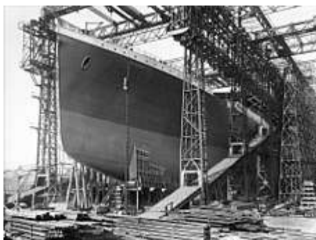
Construction in gantry, 1909–11
