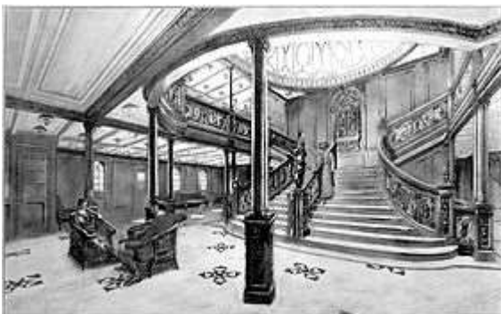
The famous Grand Staircase, which connected Boat Deck and E Deck
